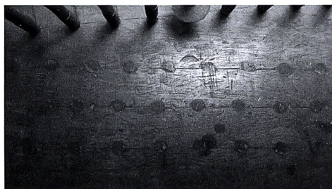
Fig 1 The wrest-plank showing the 3 rows of original wrest pin holes, subsequently plugged.]
